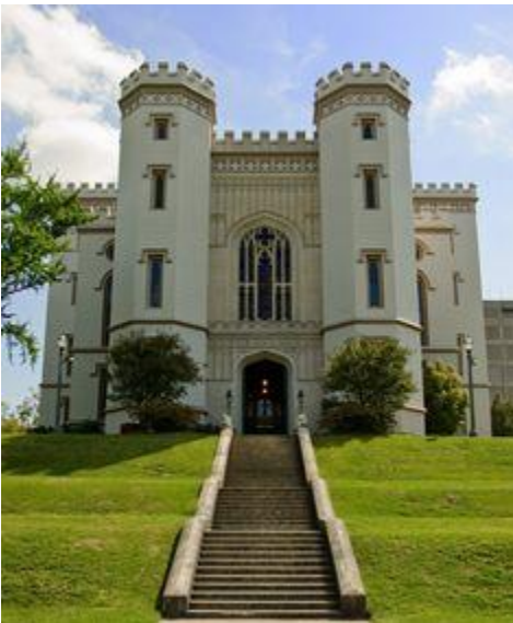
Louisiana's Old State Capitol, built 1847-52
